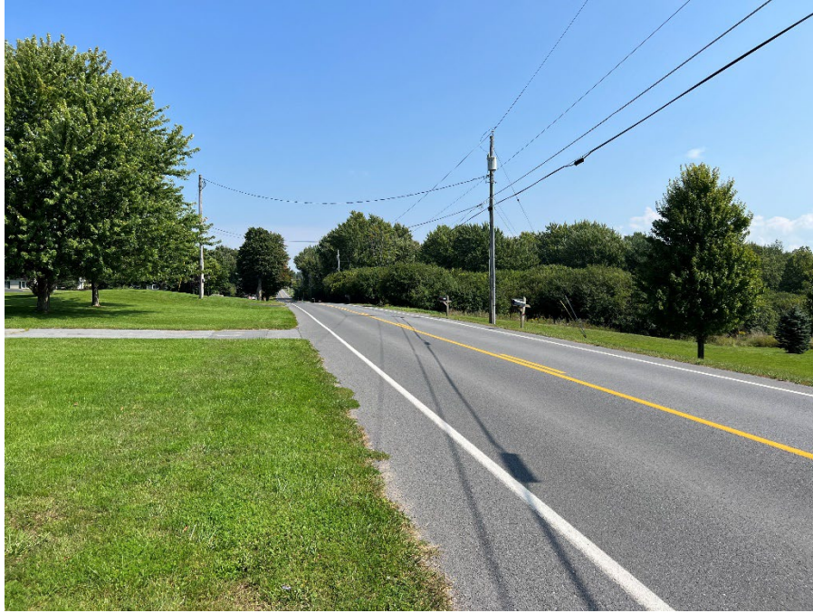
LOOKING NORTHEAST ALONG IVES STREET FROM FLUSHING HYDRANT
