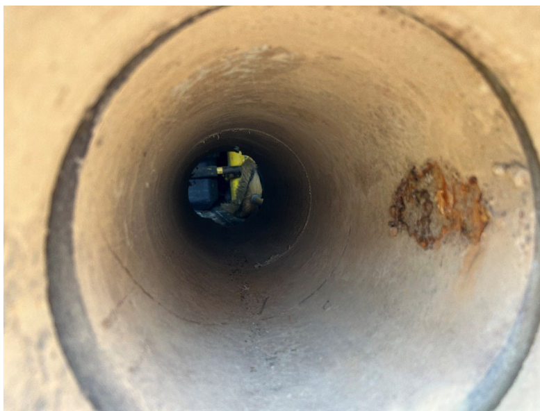
INTERIOR OF WATER PIPE
