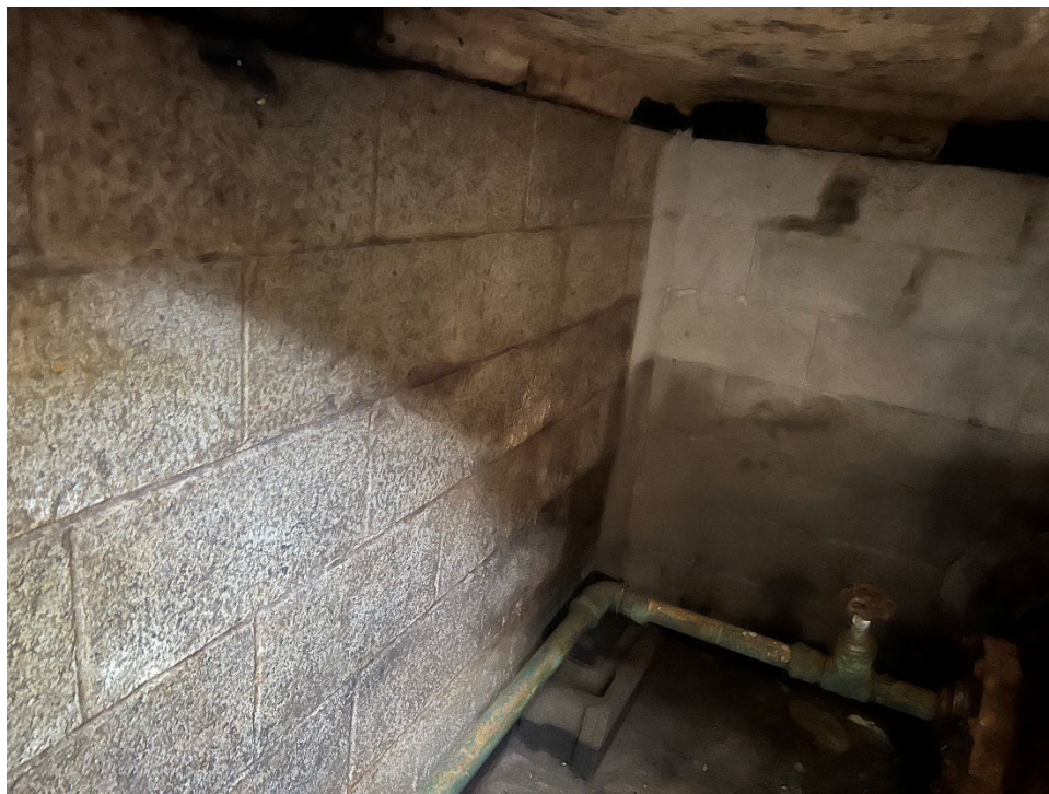
INTERIOR WALLS OF METER PIT
